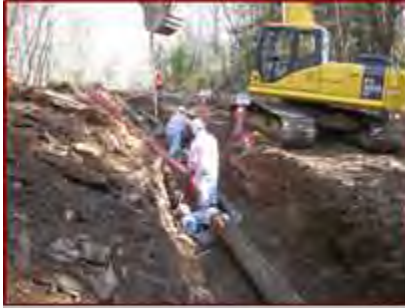
Navy Jet Fuel Pipeline Removal Harpswell & Brunswick, ME
