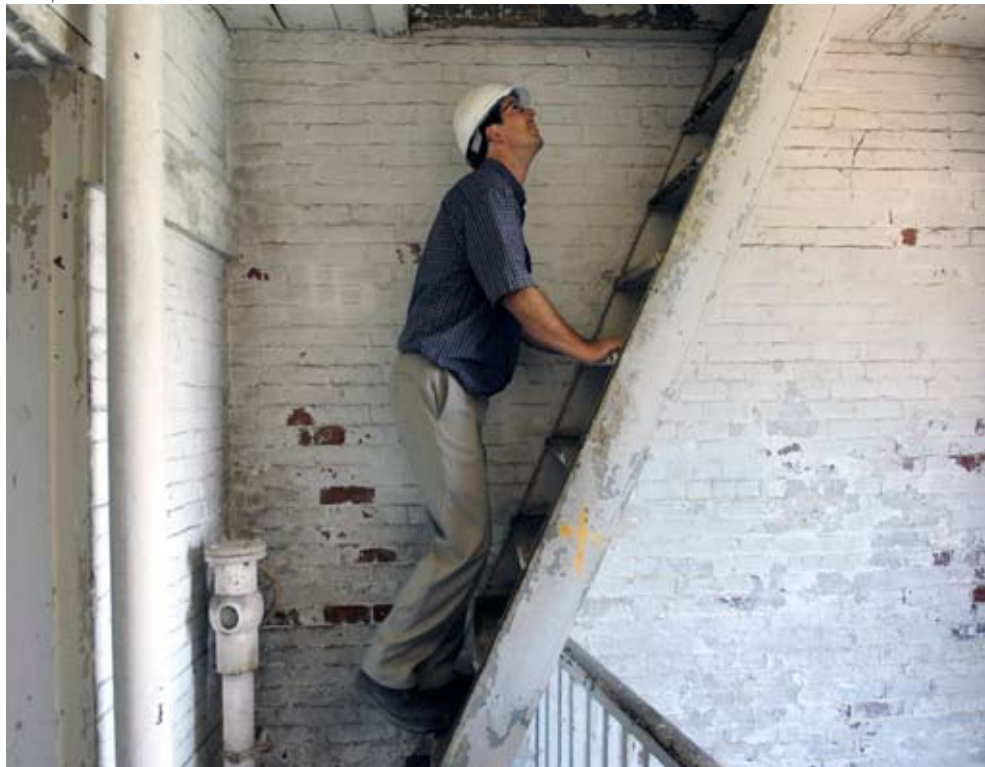
The first stage: Rip Patten, shown here climbing to the bell tower of the North Berwick Woolen Mill, checks for asbestos and other contaminants at former industrial sites before they can be redeveloped
