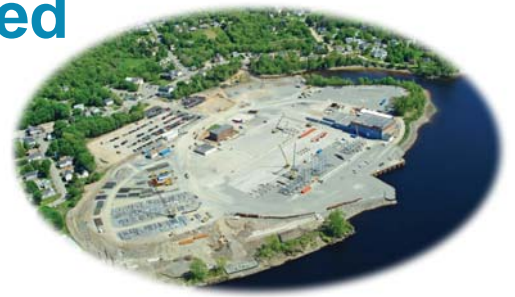
An aerial view of the redeveloped property, with module construction underway.
